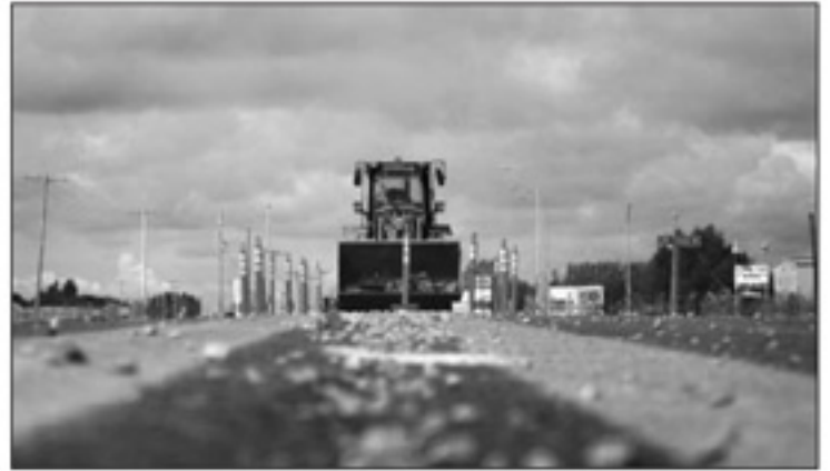
Work continues on the truck route along Highway 16
