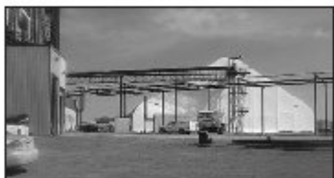
P & H has had a presence in Yorkton for over 6 decades. The newly installed grain storage bunker is a concept new to the prairies.
